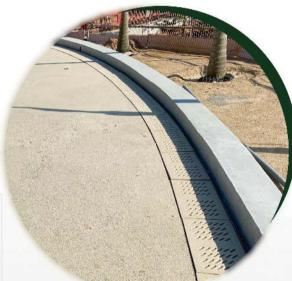
Moulded FRP gratings are in form of regular mesh or slot types. They are formed in large metal moulds with hand-laid glass fibres as reinforcement and resins as matrix.
